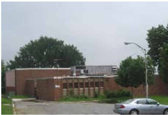
Recreation Center, south side
